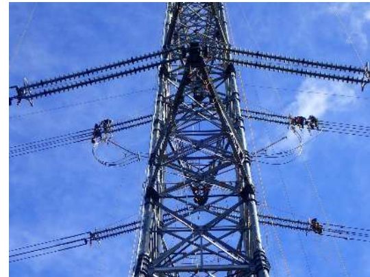
C. 架線工事 (No.86)
